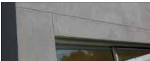
Figure 2.7.1 Neat finish of horizontal joints
