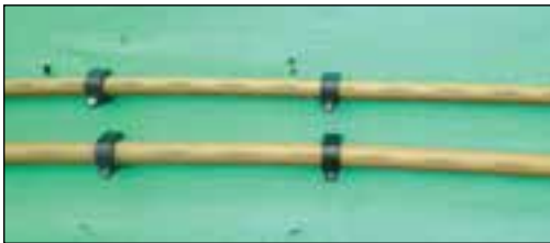
Figure 2.6.1 Installed piping services prior to the installation of Hebel PowerPanel 50
